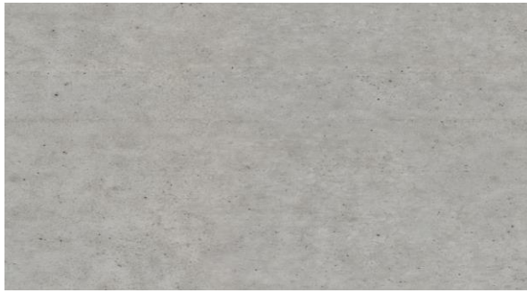
Cast in place reinforced form concrete
