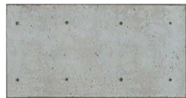
Cast in place reinforced form concrete
