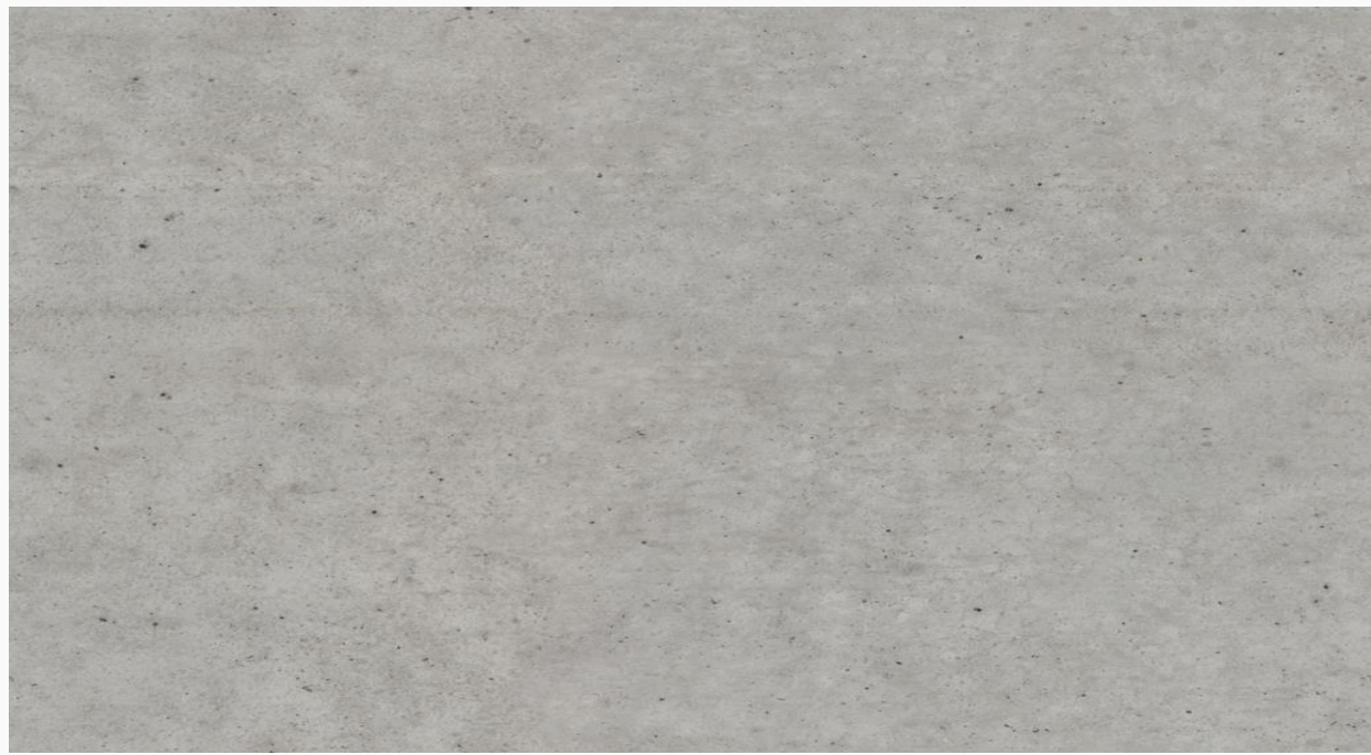
Cast in place reinforced form concrete
