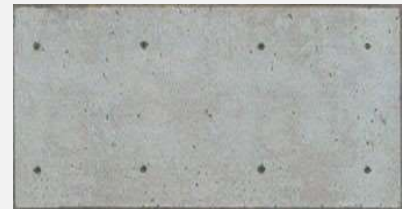
Cast in place reinforced form concrete
