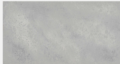
Cast in place reinforce concrete
